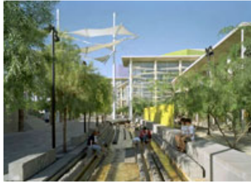
Figure 12: Arizona's Mesa Arts Center inspires the channel west of Ackerman.
