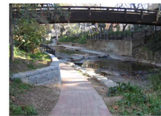
Daylighting project cuts through San Luis Obispo.
